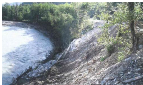
Figure 1 - Destruction of the section of the road A-149 Adler - Krasnaya Polyana, km 19+500
